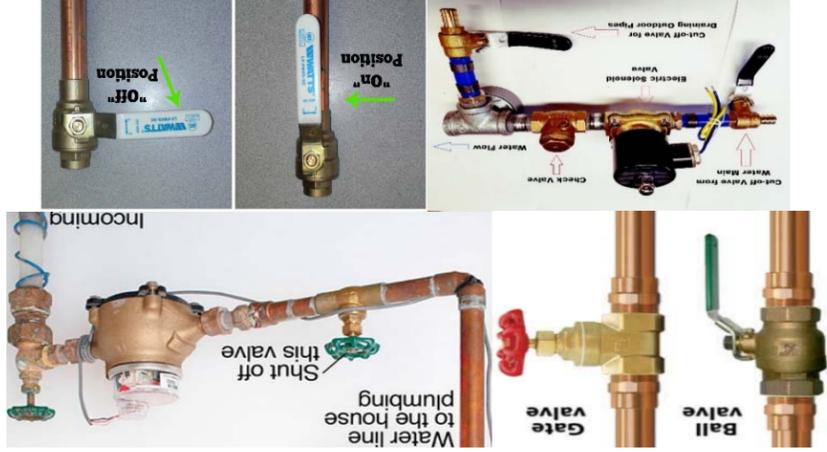
Your house may also have a solenoid switch which is an electronic switch used to turn water on and off. They are also used as access to drain valves for winterizing home. It is important to know if you have one, where it is and how / what it operates. If this switch is left on, it can continuously run water into a drain valve causing unexpected high usage.
